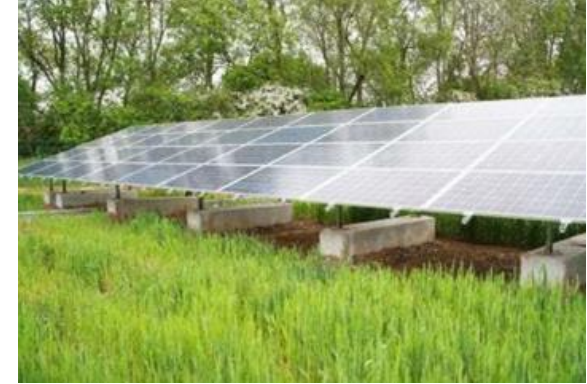
Panels with Concrete Feet
